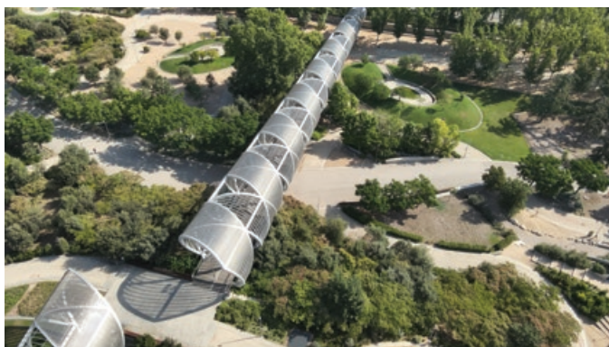
The Perrault footbridge is an iconic landmark of the Madrid Río, linking the districts of Arganzuela and Carabanchel. It was inaugurated in March 2011. Image: Madrid City Council
